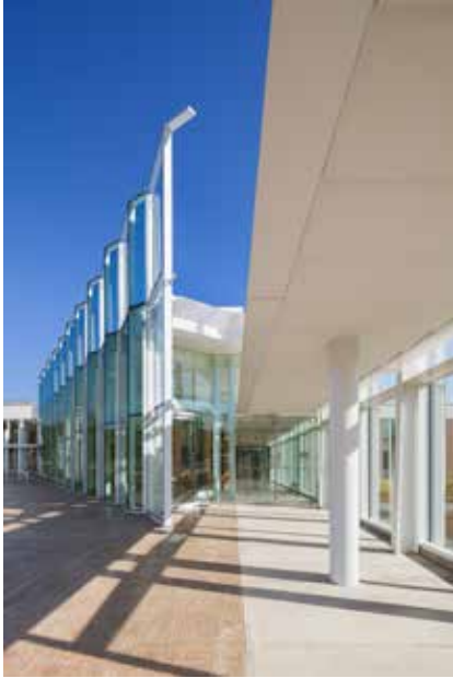
Main entrance detail
