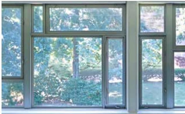
The new glazing system uses only two typical window configurations. However, through mirroring and combinations of these two units a unique appearance was obtained for each individual classroom reducing the sense of uniformity in the existing repetitive building layout.
